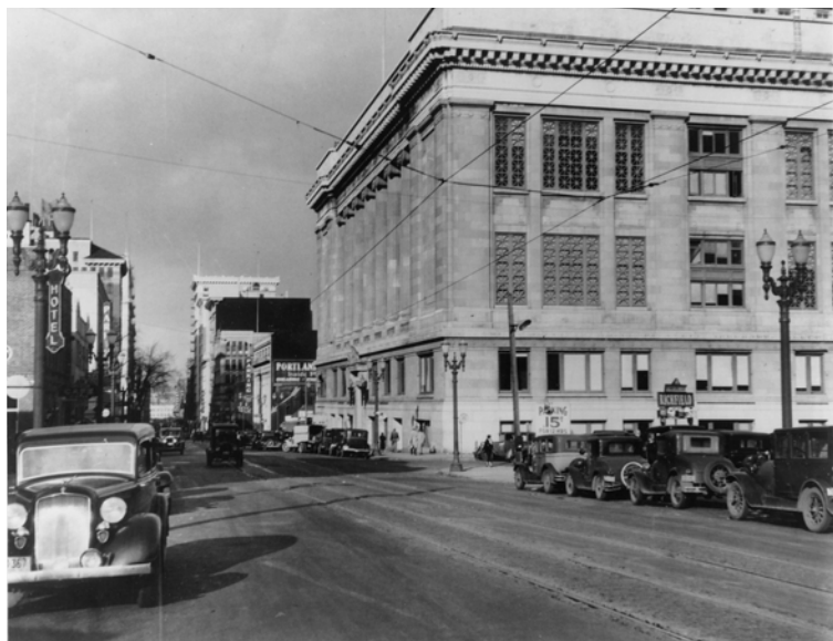
Multnomah County Courthouse as it appeared in 1934
