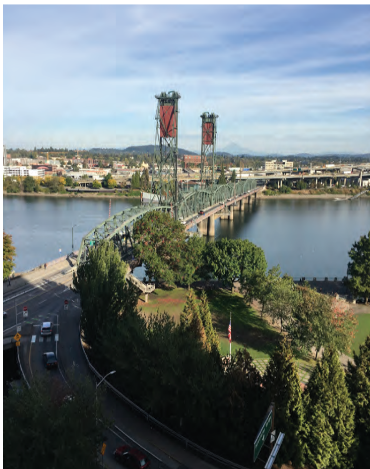
The public spaces will enjoy a spectacular view of the Hawthorne Bridge and Willamette River
